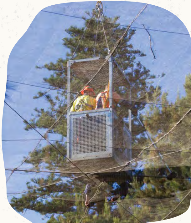
The netting of the Australian Wetlands was repaired.
