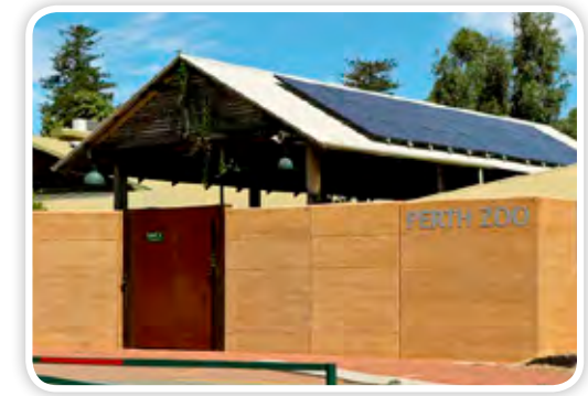
Solar power at Perth Zoo
